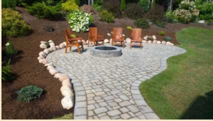
New paver patio with fire pit, new beds and sods around
