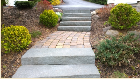
New steps, paver walkway and surrounding shrub beds
